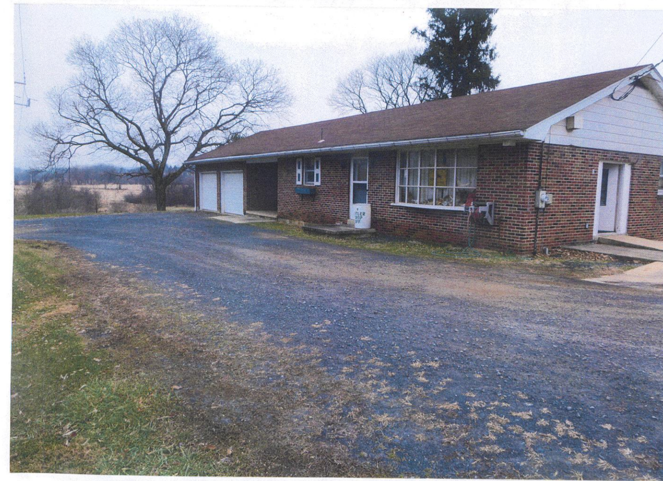
PICTURE OF BUILDING (SOUTH SIDE)
