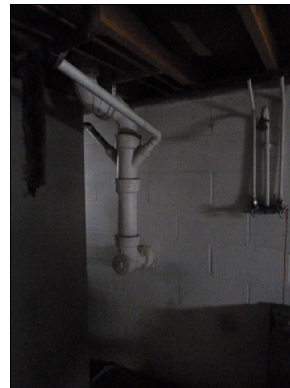
PHOTOGRAPH OF EXISTING SEWER LATERAL NO SCALE
